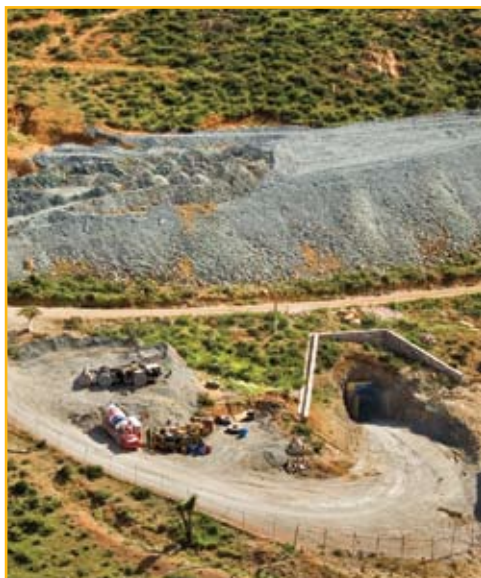
Vehicle access to the Cozamin mine is through the San Ernesto portal.
