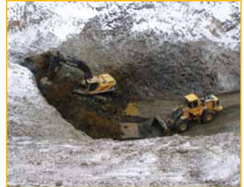
Portal preparations for the bulk sample drift at Stora Sahavaara, Sweden.
