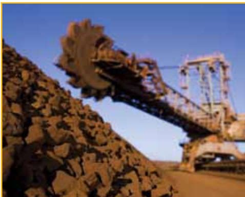
A reclaimer in action at Parker Point ship loading terminal, Rio Tinto, Dampier Port, Australia.
